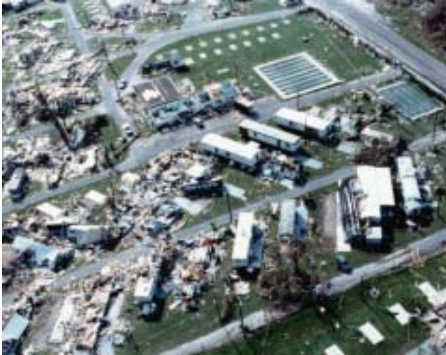
Mobile homes and portable structures were the first to fall under the wrath of Hurricane Andrew in 1992. Photo courtesy of the State Archives of Florida, Florida Department of State, Photographic Collection.
